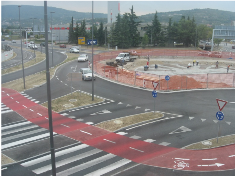
Figure 8. The first Slovenian turbo roundabout – under construction; city Koper, 2008
