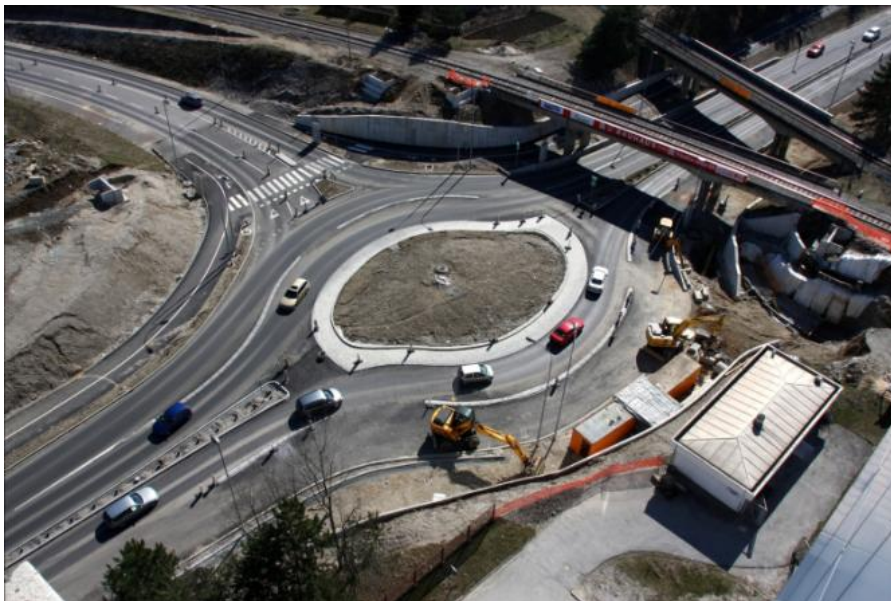
Figure 9. The second Slovenian Turbo Roundabout – under construction; city Maribor, 2009
