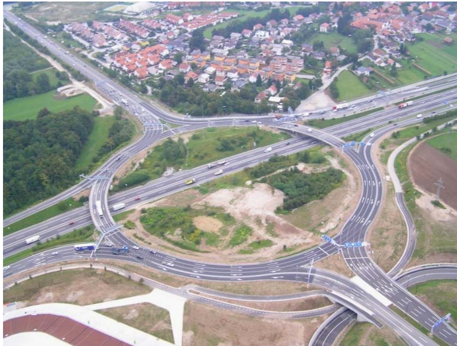
Figure 3. The first Slovenian traffic-lighted turbo roundabout in Ljubljana: equipped with traffic lights on each entry and on inner lanes (dynamic controlled, with in-pavement detectors)
