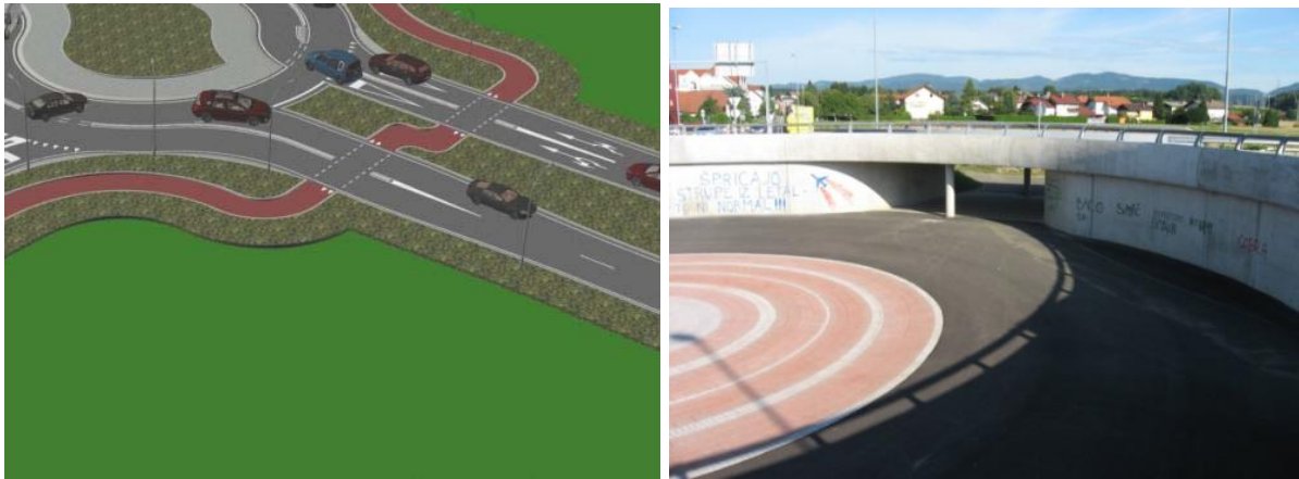
Figure 6. Deviated position of the pedestrian and cycle crossing (left) and leading non-motorized traffic participants in different level (right)
