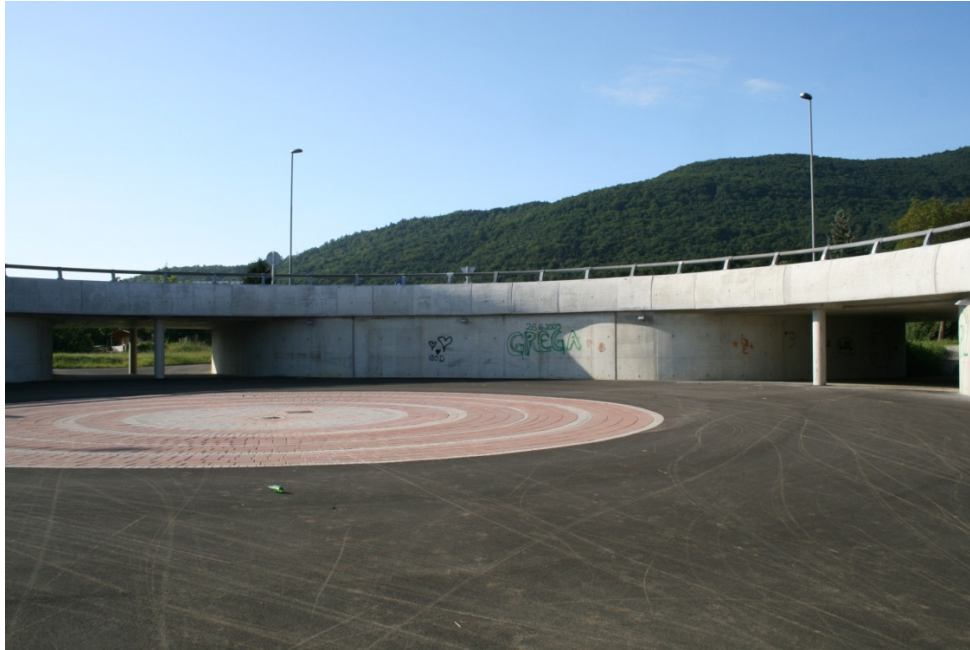
Figure 20. Turbo Roundabout M3 “Lackova” in Maribor: underpass for pedestrians and cyclists
