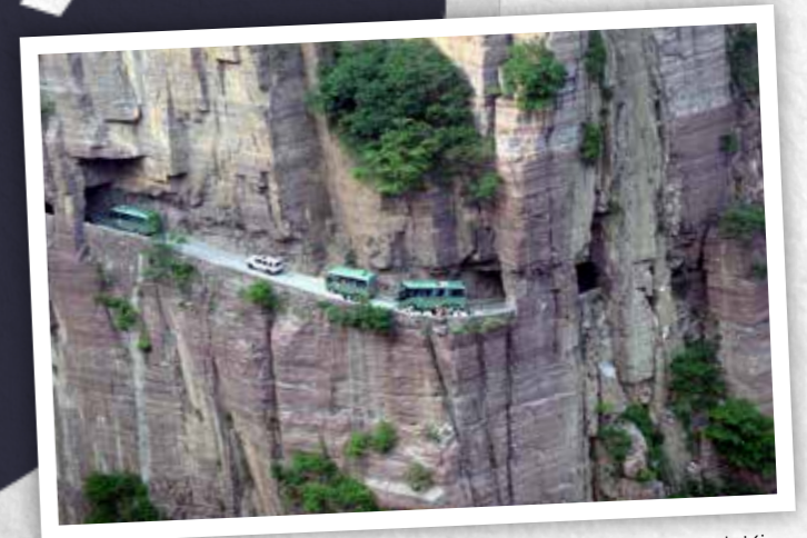
Guoliang Tunnel, Kina
